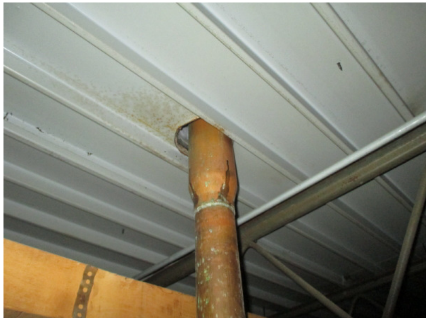
Plumbing stack/vent pipe
