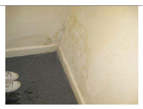
This probably only occurs during heavy rains. Repair/replacement of leaky gutters and downspouts and (if necessary) re-grading are recommended, and may fully correct this. If not, waterproofing and/or replacement of finished walls using moisture-resistant materials may be necessary.
