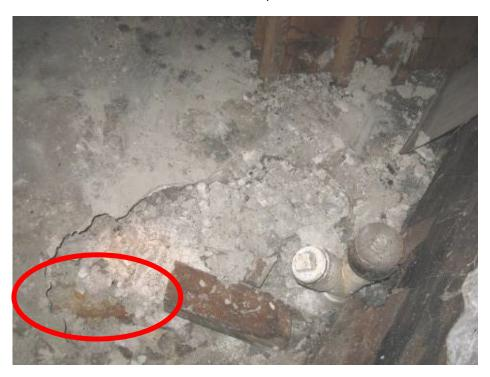
Some sections of this pipe had been repaired with new PVC piping. It appeared likely the remainder of the line would need to be replaced in the near future. It may be best to do this when extensive supply line updates are done.
